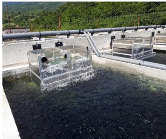
Figure 3. Oxygen-box with lifting pump at the trout farm of Tropic Fishery in Bosnia and Herzegovina (foto N. Savić, 2020)
