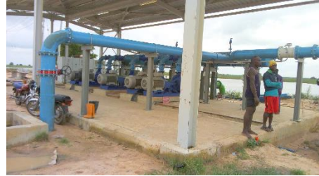
Fig. 12. A completed drainage pump lifting water above the dyke out of the field
