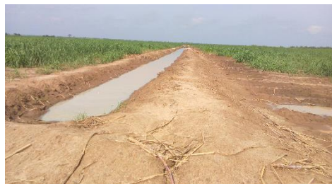
Fig. 10. An earth canal for surface irrigation
