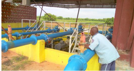
Fig. 11. Pump station for surface irrigation station
