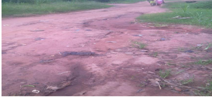
Plate 7: Erosion at site G
