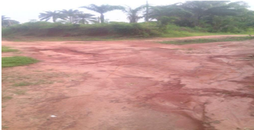
Plate 4: Erosion at site D
