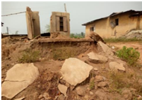
Fig. 1.1. Building structure affected by blasting in the AC Source: Field survey (2024).
